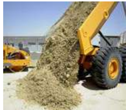
BACK FILLING - GATCH MATERIAL
